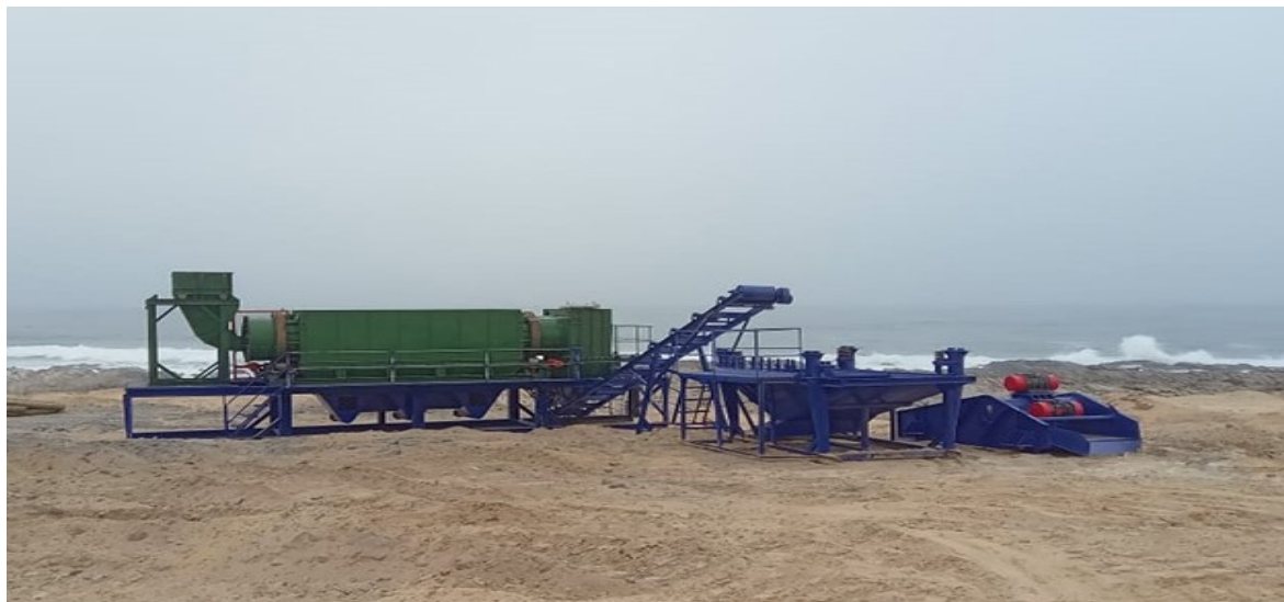
April 2024 - Trommel screen, screener/scalper conveyors and feed bins installed. Source: Company
